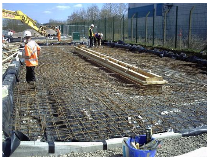
Figure 1 Membrane installation below steel reinforcement is subject to high puncture forces
